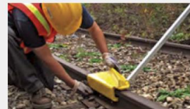
Track management staff placing a derail on railway track.
